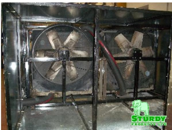
Photo 3 The two heat exchangers mounted in the ducting
